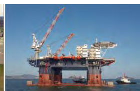
Offshore oil platform
