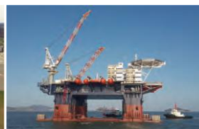
Offshore oil platform
